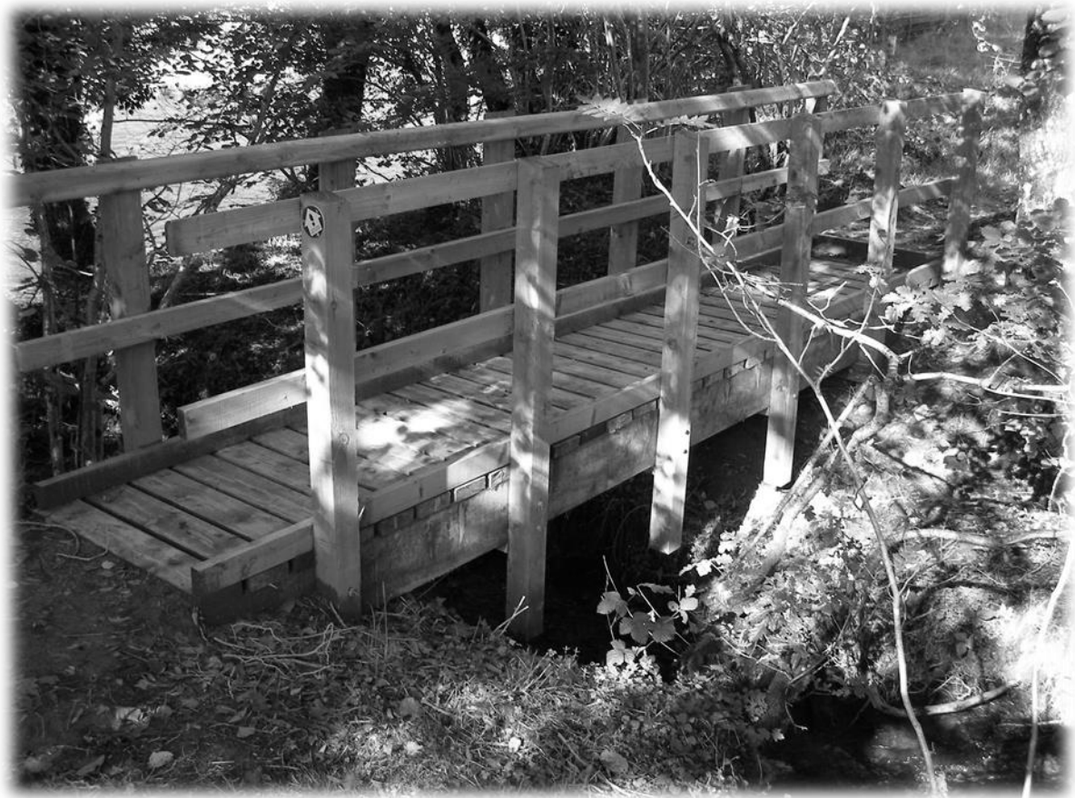
Timber Footbridge, Llanfair ar y Bryn
